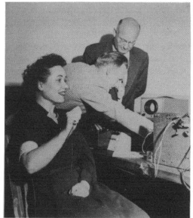
Fig. 3 - Determination of perception current on the hands.
